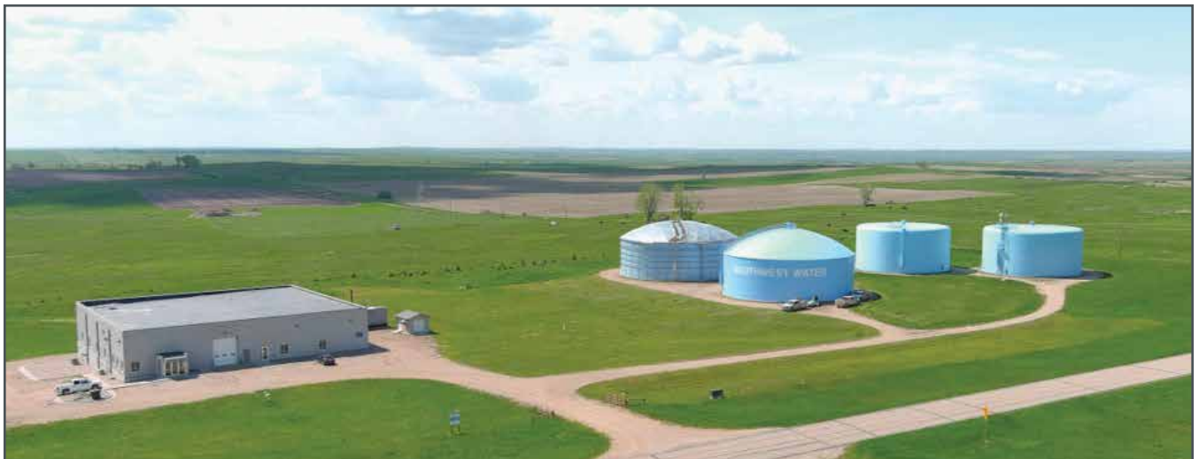
SWA Water Treatment Plant.
