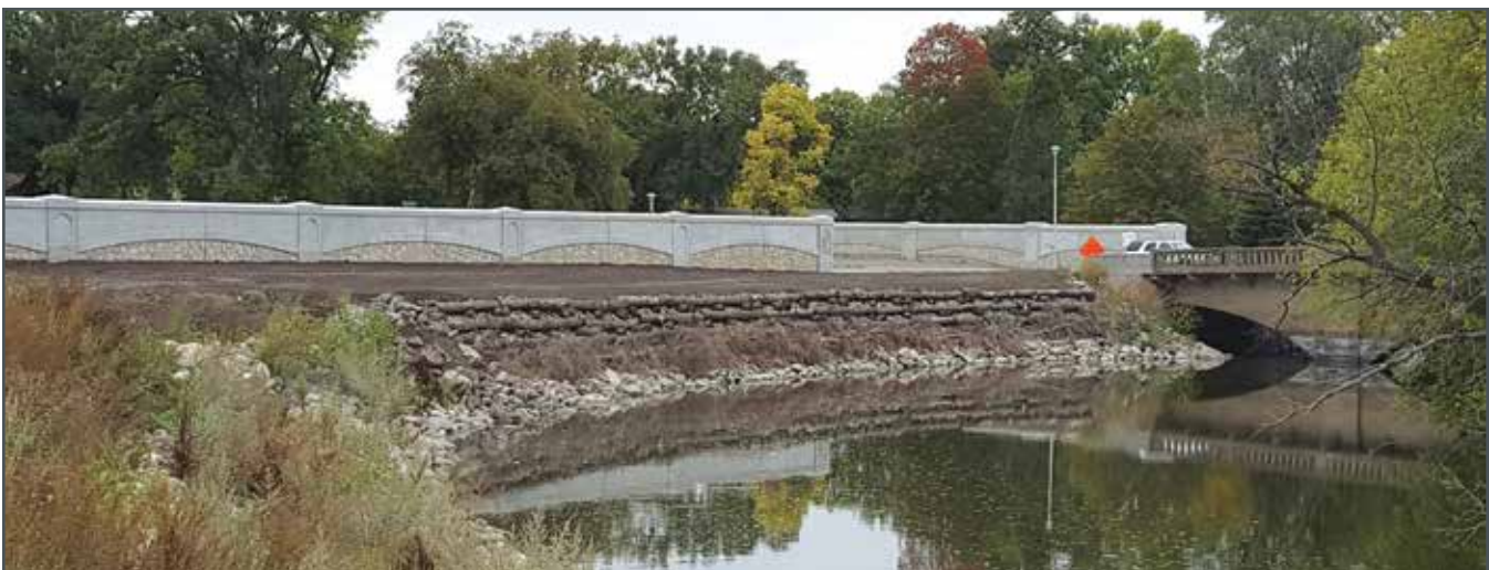
Valley City permanent flood protection at 4th Street SW.
