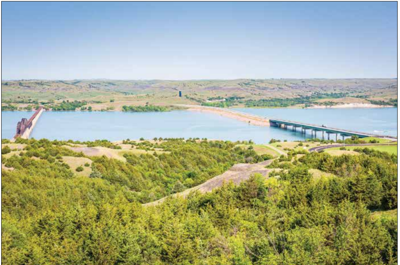
Chamberlain Bridge and Lewis and Clark Memorial Bridge in South Dakota.
