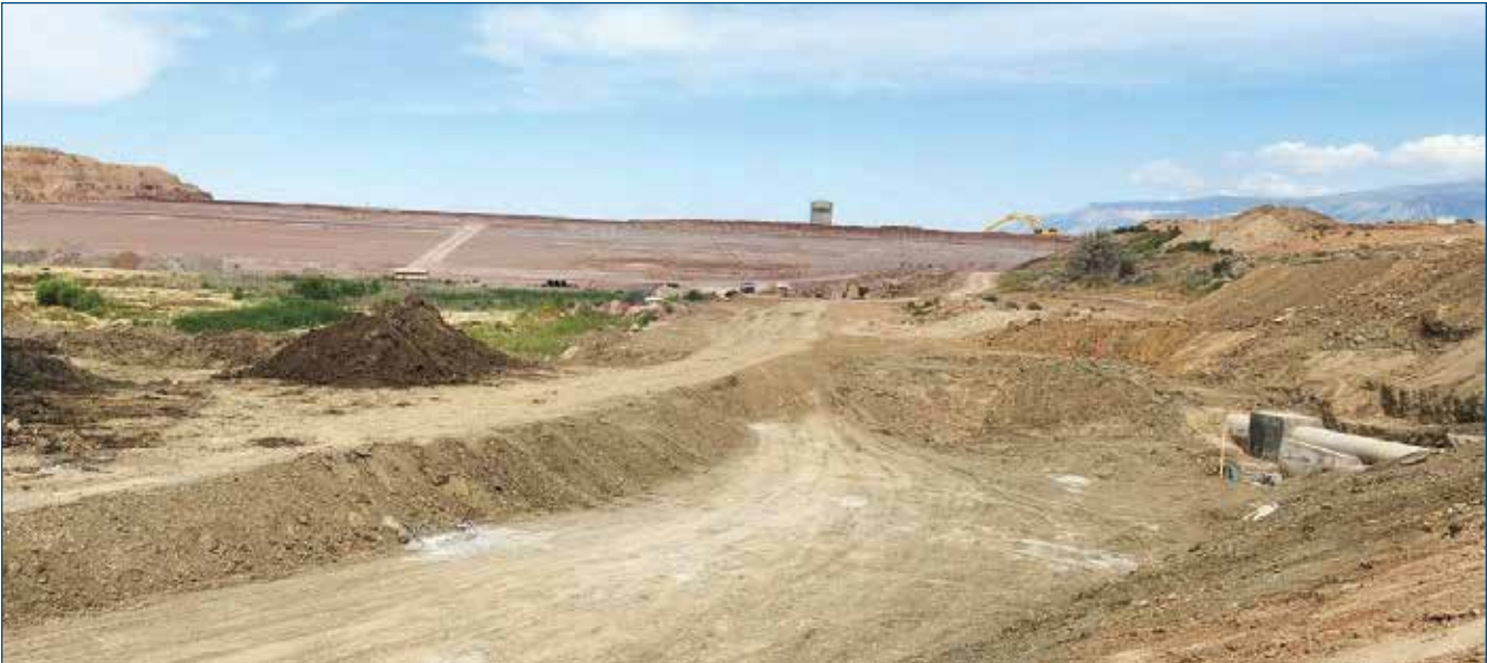
Leavitt Reservoir Construction July 2025. Photo credit: Bill Brewer, WWDO staff
